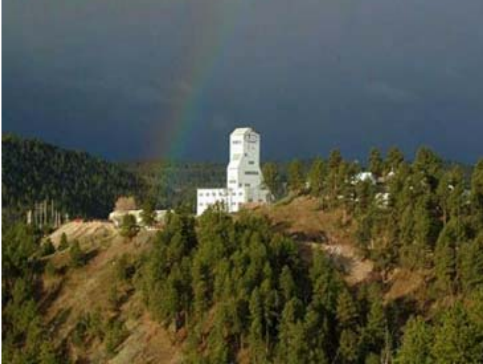
The Ross headframe, Homestake Mine. Scientific access to the three levels of the proposed National Underground Science and Engineering Laboratory, on the 4850, 7400, and 8000 ft levels, will be via the Ross hoist and No. 6 Winze.
